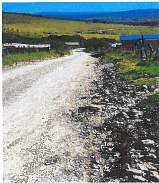
The surfacing of gravel is complete however the v drains and storm water pipes are not installed.
