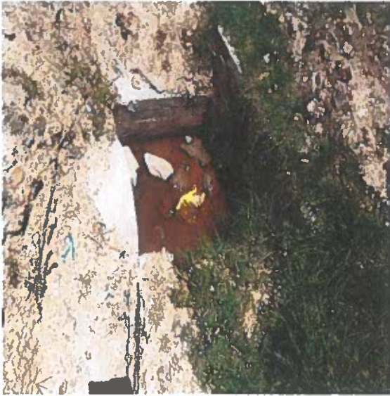
Blockage of existing storm water drainages
