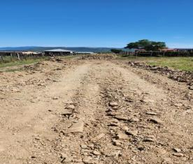
The road has been shaped and graveled. Bedding laid Second course will be added. Subsoil drain and stone pitching will be installed.
